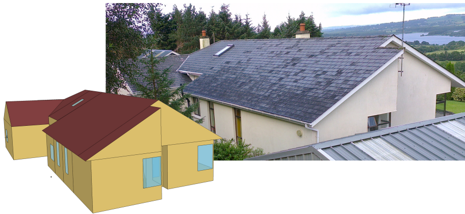
Figure 1: Test bed house and EnergyPlus model
